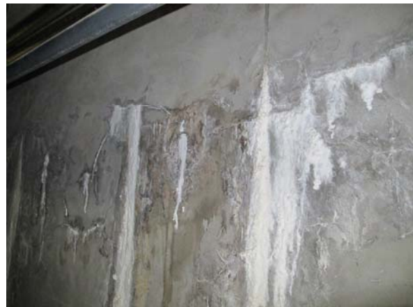
Visible damages to the concrete (cracks, effluorescence, steel corrosion products) due to ingress of water loaded with calcium hypochlorite into the concrete structure of the pools of the Zwembad Overbosch.
