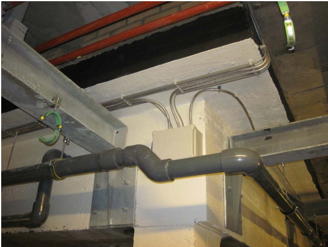
Acrylic cover coating (Sikkens Alphatex IQ) on the CAST 3+ Composite Anode installed on the outside walls of the swimming pools
