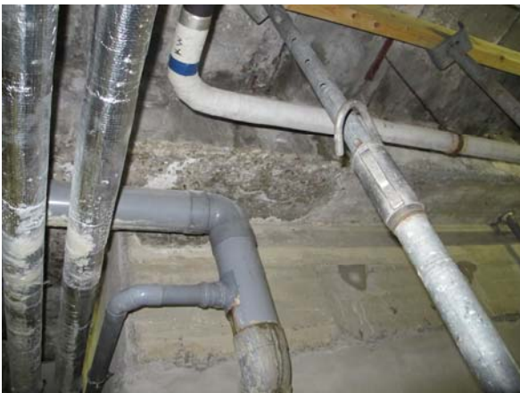
Visible damages to the concrete (cracks, effluorescence, steel corrosion products) due to ingress of water loaded with calcium hypochlorite into the concrete structure of the pools of the Zwembad Overbosch.
