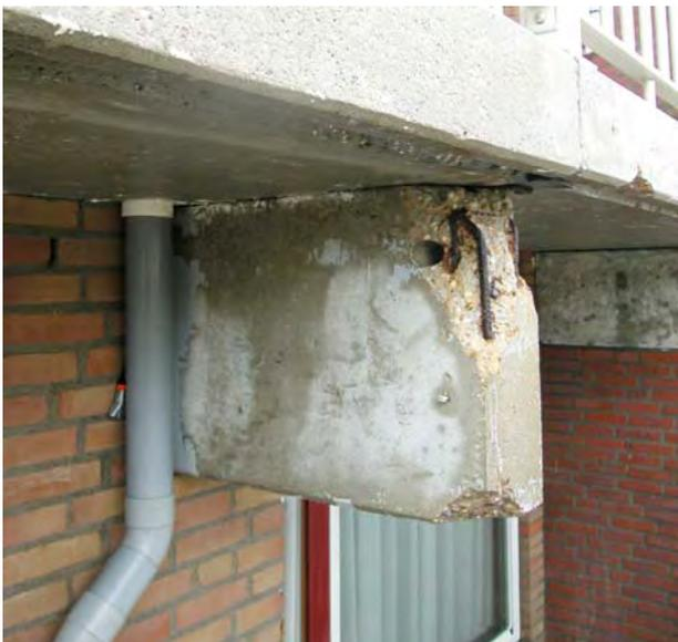
Figure 2: Spalling and local destruction of the concrete cover of supporting beams, severe loss of cross section of steel rebars due to steel rebar corrosion.
