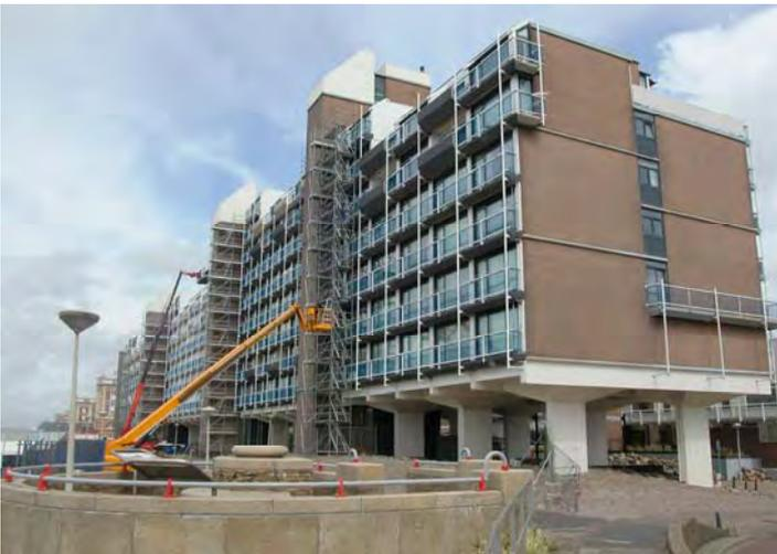
Figure 5: Installation of the CAST<sup>+</sup> composite anode system on apartment buildings in Scheveningen 2008.
