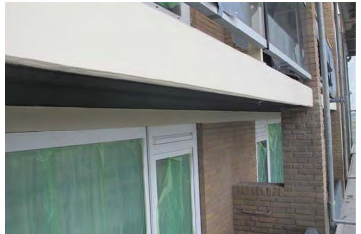
Figure 15: Application of a white top coat after the installation of the CAST<sup>3+</sup> system.
