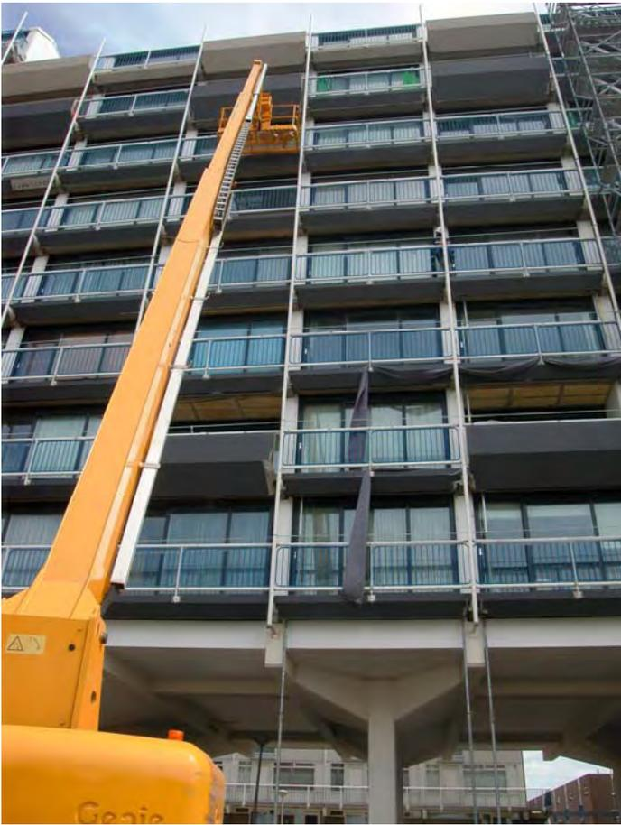
Figure 8: Application of the CAST+ composite paint on balconies, roof decks and balustrades (paint with anthracite colour).
