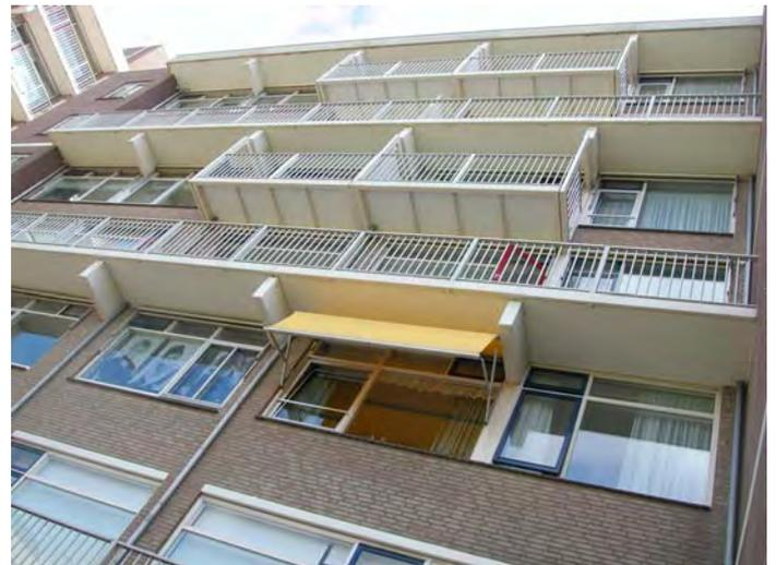
Figure 11: View on the apartment building after application of the CAST+ system and after application of white acrylic cover coating.
