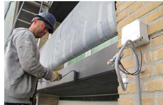
Figure 13: Balustrades and underside of balcony, coated with the CAST<sup>3+</sup> composite anode paint.
