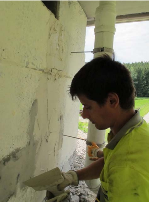
Application of the EZA binder before applying the zinc mesh
