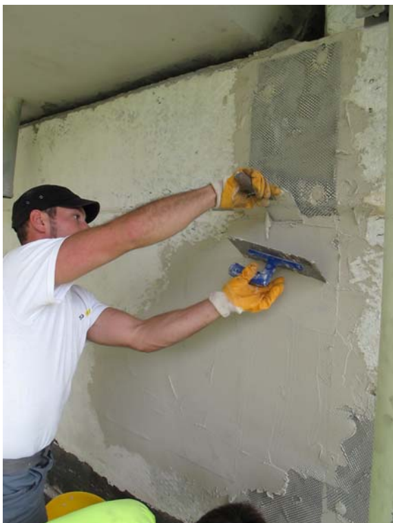
Application of the EZA binder before applying the zinc mesh
