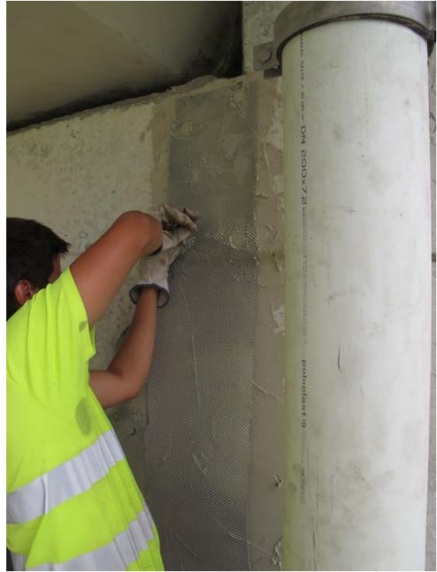
Application of the new zinc mesh and fixation with dowel pins
