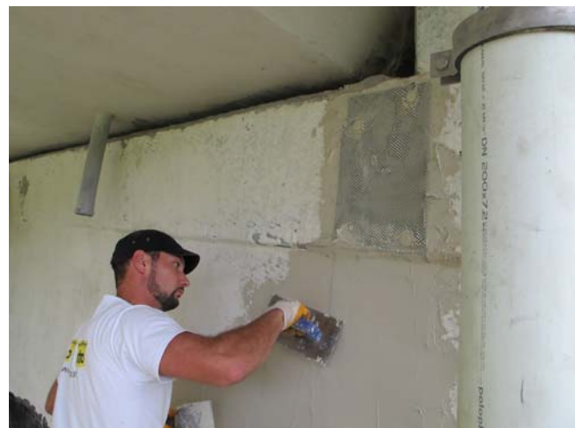
Embedding the zinc mesh with the EZA binder
