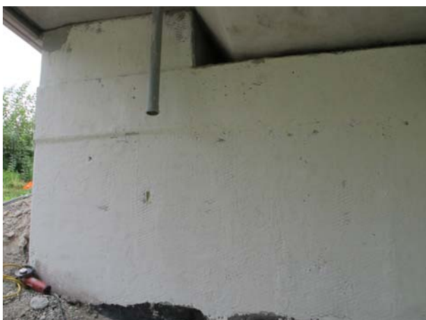
Detail after sandblasting: abutment hillside (left), middle part of abutment (right)
