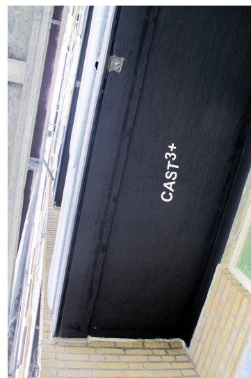
The CAST 3+ composite anode was applied on the soffit of the balconies
