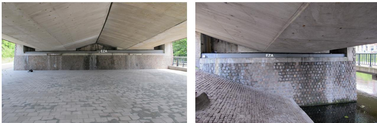
**Fig. 6** EZA installed on the beams supporting the bearings of abutments of the Hubertus viaduct in The Hague
