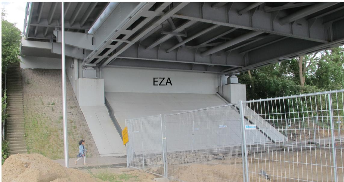
*Fig. 6 De Meerenbrug steel bridge in Utrecht with concrete abutments*
