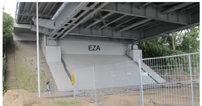
Figure 5. De Meerenbrugg steel bridge (top) in Utrecht with concrete abutments (bottom)
