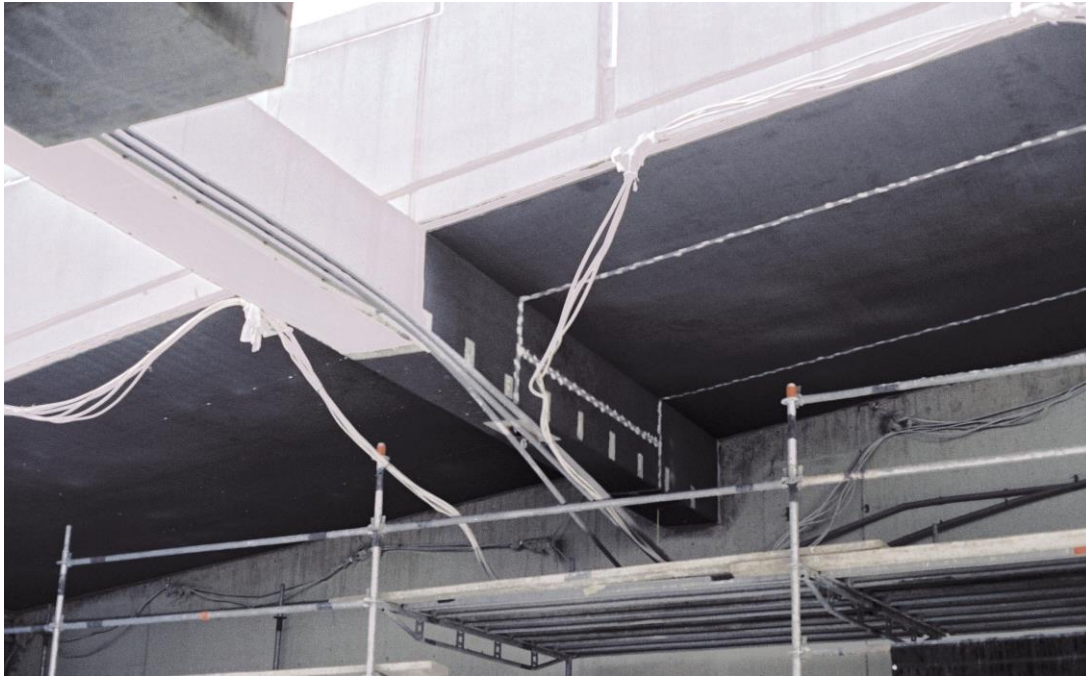
Application of Composite Anode on Parking Deck Soffits
