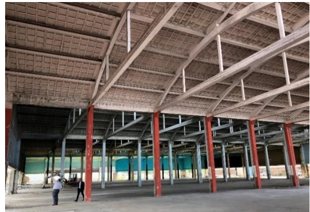
Fig. 13. Concrete elements of the main structure on the interior
