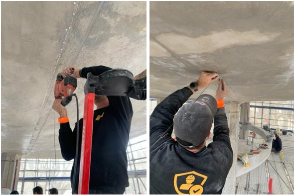
Fig. 35. Installation of one of the primary anodes.
