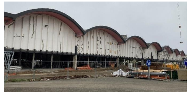
Fig. 18. Applied anode material (black conductive coating) on roof elements and ribs
