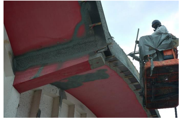
Fig. 16. Concrete repair with shotcrete at a roof element
