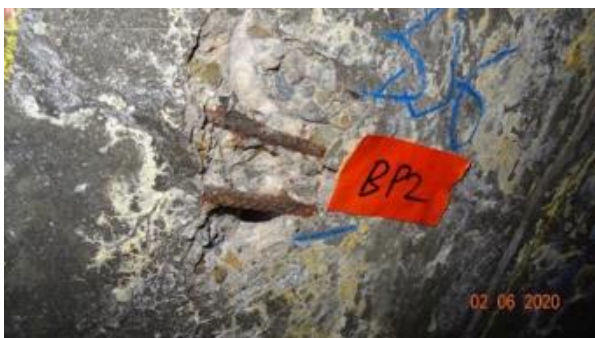
Fig. 25. Image: Exploratory Openings
