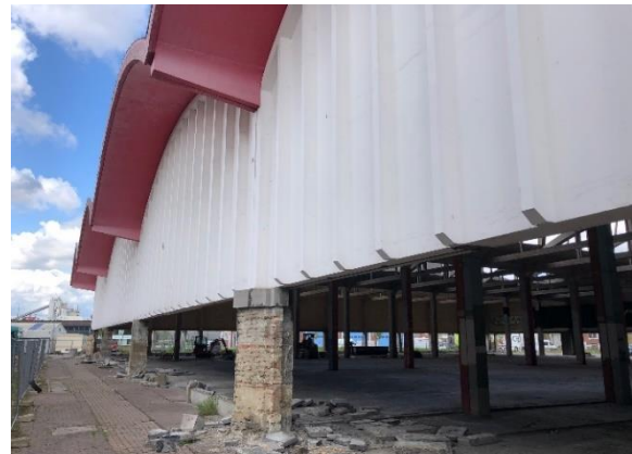
Fig. 14. Concrete elements of the main structure on the exterior
