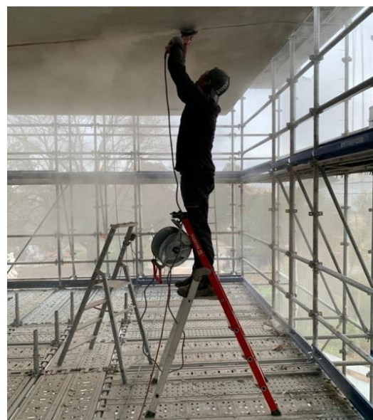
Fig. 34. Preparation of the grooves to dissimulate the XLPE/XLPE cables.
