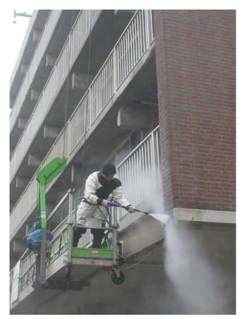
Figure 10: Concrete surface preparation and cleaning by high pressure water jetting.
