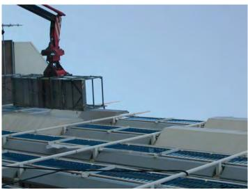
Figure 7: Cleaning of the concrete surface by high pressure water jetting.
