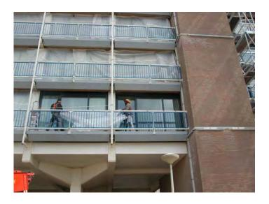
Figure 6: Covering the windows with plastic sheets before repair and installation works start.
