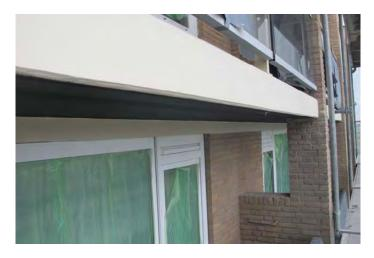
Figure 15: Application of a white top coat after the installation of the  $CAST^{3+}$  system.
