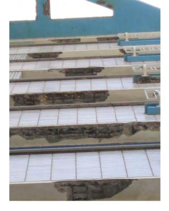
Figure 1: Spalling and disbondement of the concrete cover due to steel rebar corrosion.
