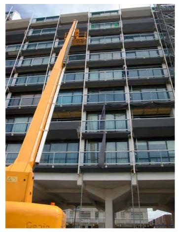
Figure 8: Application of the CAST+ composite paint on balconies, roof decks and balustrades (paint with anthracite colour).
