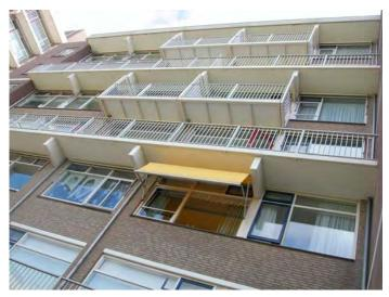
Figure 11: View on the apartment building after application of the  $CAST^+$  system and after application of white acrylic cover coating.
