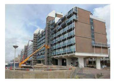
Figure 5: Installation of the CAST<sup>+</sup> composite anode system on apartment buildings in Scheveningen 2008.
