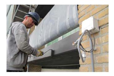
Figure 13: Balustrades and underside of balcony, coated with the  $CAST^{3+}$  composite anode paint.
