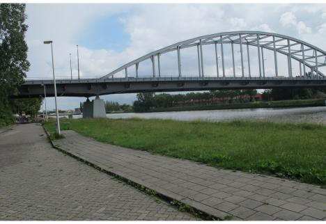
Fig. 5 De Meerenbrugg steel bridge in Utrecht with concrete abutments
