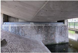
**Fig. 6** EZA installed on the beams supporting the bearings of abutments of the Hubertus viaduct in The Hague
