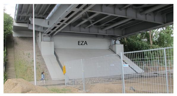
Fig. 6 De Meerenbrugg steel bridge in Utrecht with concrete abutments
