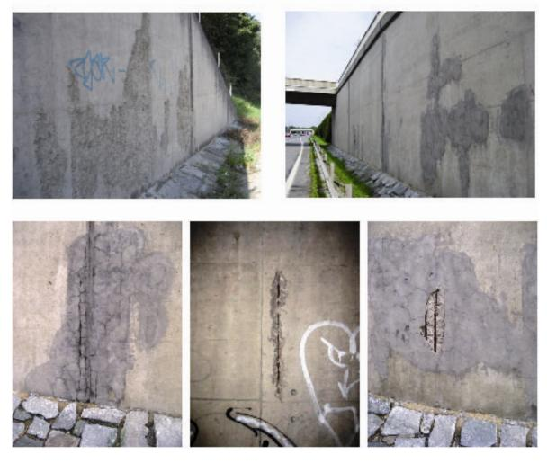
Figure 3: Visible damages to the sustaining wall of the bridge B2134.
