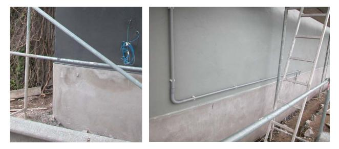
Figure 12: Installation of the titanium ribbon mesh anode on the sustaining wall above and below the ground line, embedded into shotcrete, left picture zone 1. B2134; right picture zone 4, B2136.
