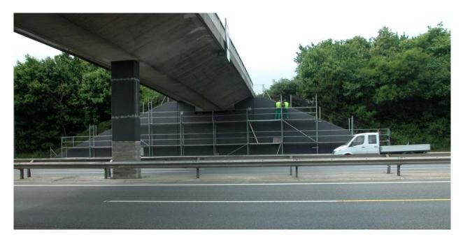
Figure 8: Installation of the CAS-Composite Anode B2134: bridge column – zone 3, CAS-CNP primary anode on  $1^{st}$  layer of CAS-T<sup>+</sup> coating; abutment – zone 2, second layer of CAS-T<sup>+</sup> coating embedding the CAS-CNP primary anode.
