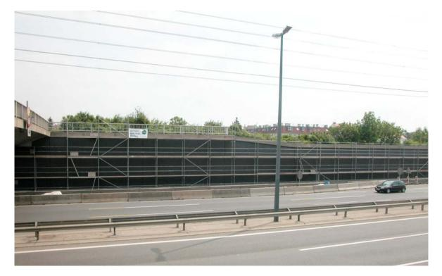
Figure 7: Installation of the CAS-Composite Anode in Zone 1 (sustaining wall, B2134 RF Stockerau) –  $1^{st}$  layer of CAS-T<sup>+</sup> coating.
