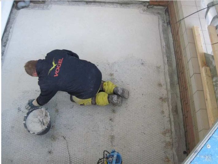
Embedding the zinc mesh into the TASC-EZA
